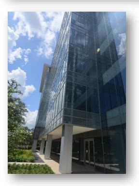
Wildwood consists of an eight-story, 211,760 SF, core and shell office building constructed of a concrete frame with curtainwall cladding, and a 240,182 SF, five-story, precast parking garage. This project was awarded **LEED** Silver Certification for the core and shell.
