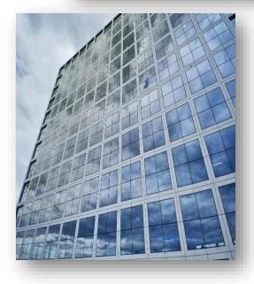
The project is a 14-story office building in the Legacy West Corporate Development in Frisco, The building features large, 15-foot Texas. square Accunit Fixed Windows in surrounding aluminum clad openings. Each window spans the full floor height divided into four equal square glass panels.
