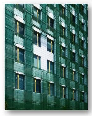
The FBI facility is an 8-story concrete building in Houston. The design incorporates Patriot Blast Resistant Fixed Window openings in the exterior walls. An aluminum lattice has also been added in front of the windows and adjacent walls that retains blue-green laminate glass covering the building's exterior façade.
